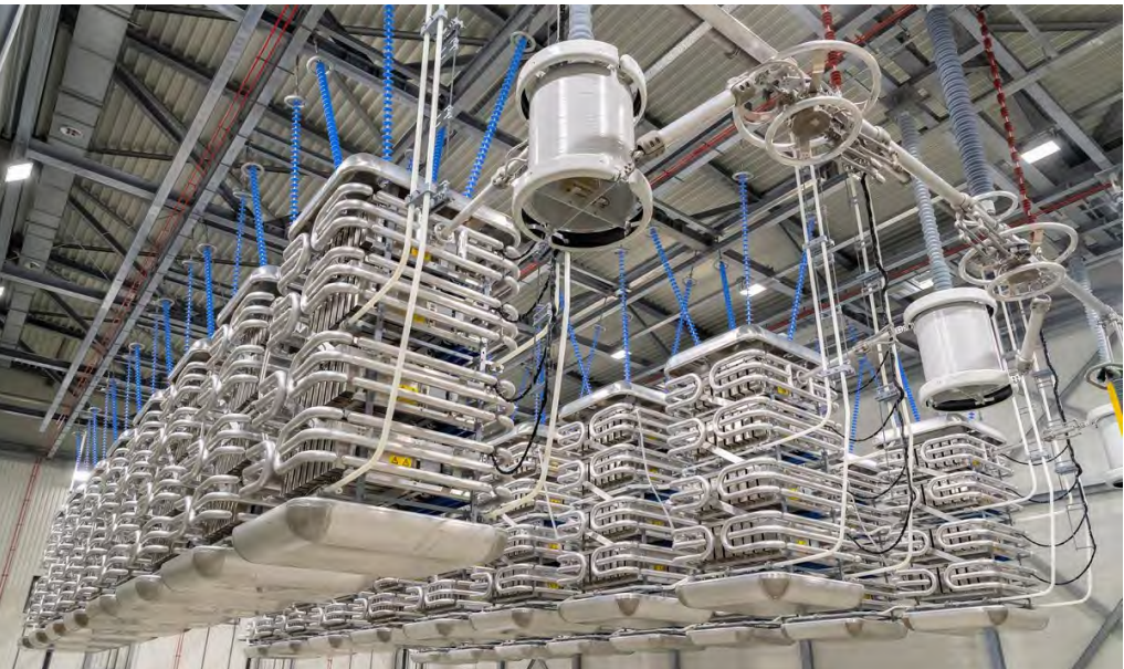
NordLink Interior view of the Valve Hall
